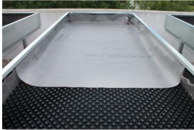
Figure 14. Drainage elements NativeScapeGR project
